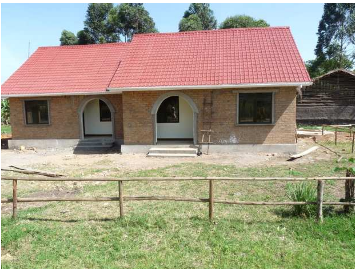
First permanent classroom building on the "America" campus of Mustard Seed. Built with interlocking stabilized soil blocks molded on the site
